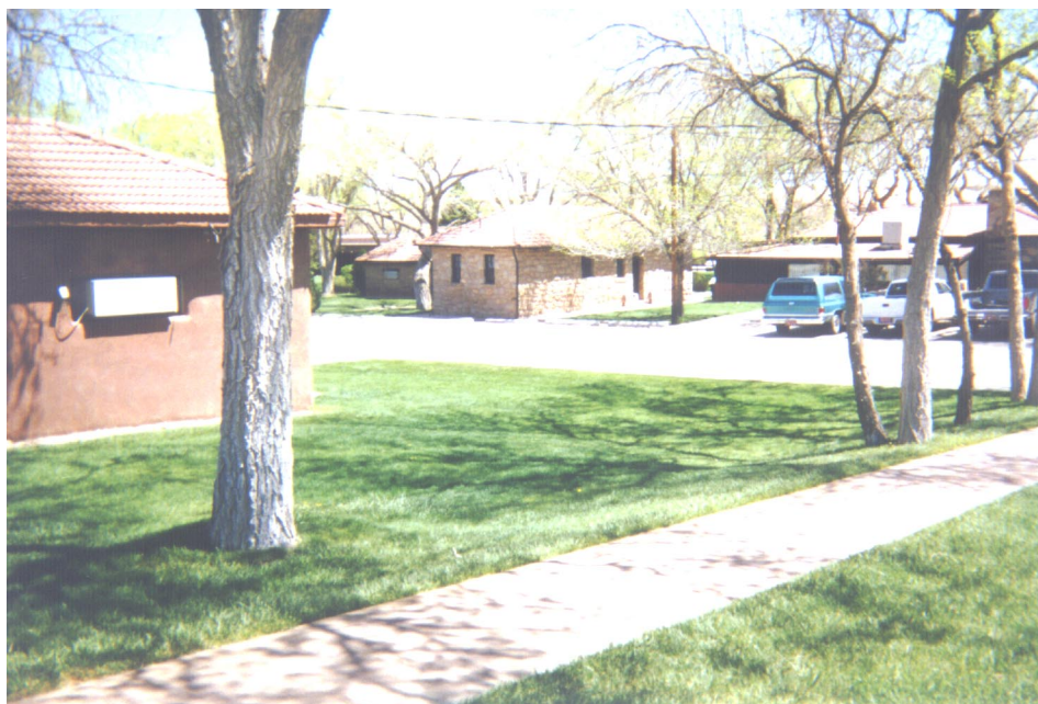
Figure II.3: Well-Maintained Lodge Buildings and Grounds at Canyon de Chelly National Monument
