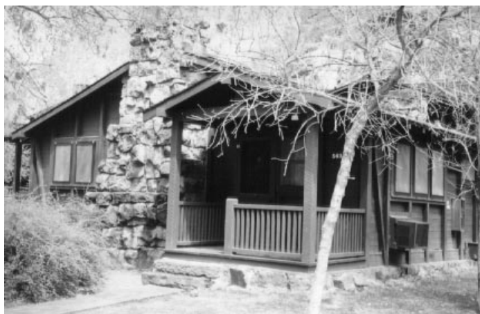
Figure II.11: Well-Maintained Cabins and Motel at Zion National Park
