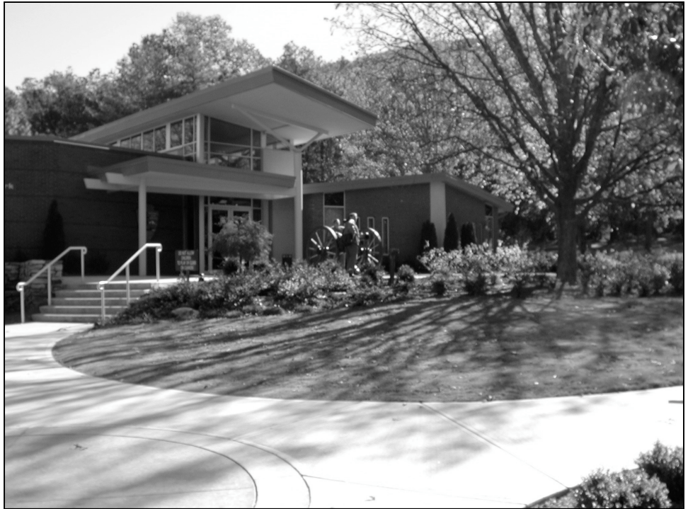
Figure 4: Addition to Kennesaw Mountain National Battlefield Park Visitor Center
