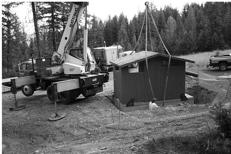
Figure 7: Installation of Public Toilet at the Treasure Interface Pilot Project, Kootenai National Forest
