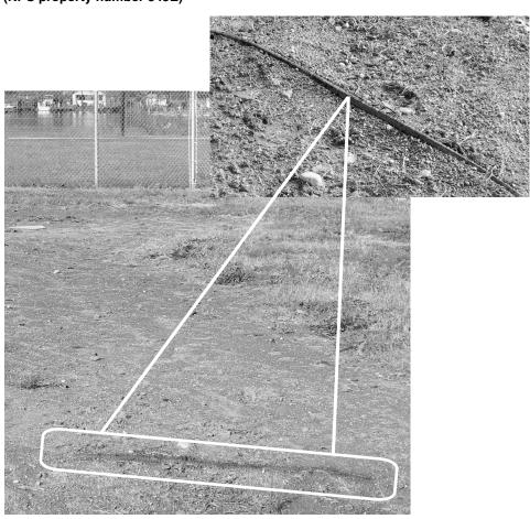
Figure 13: Exposed Metal Reinforcement Bar on a Baseball Field in Anacostia Park (NPS property number 343E)
