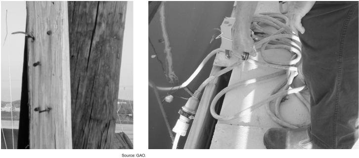
Note: The photo on the left shows exposed, rusty nails on a dock piling. The photo on the right shows an electrical cord hanging close to the water.
