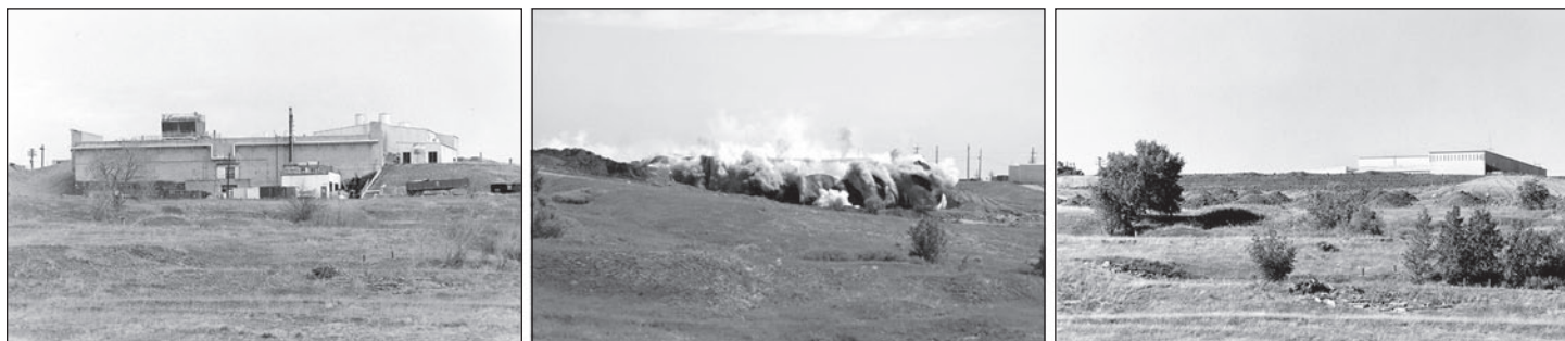
Figure 3: Use of Explosives in the Demolition of Rocky Flats' Building 881
