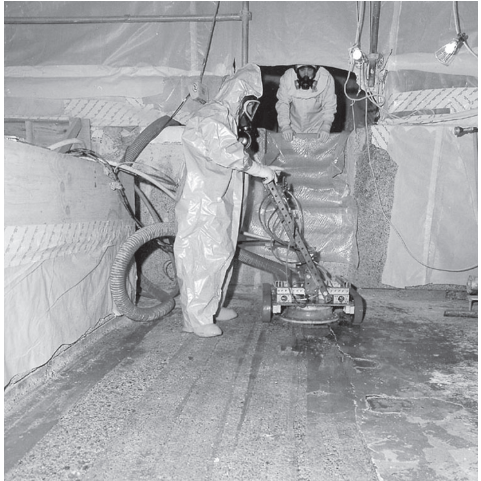
Figure 15: Hydrolase System at Work Removing Contaminated Paint and Underlying Surface Contamination
