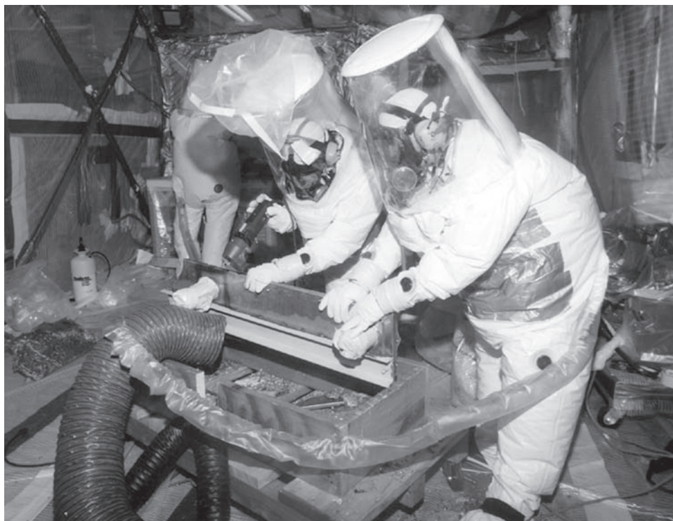
Figure 1: Workers in Protective Suits Cut Plutonium-Contaminated Equipment
