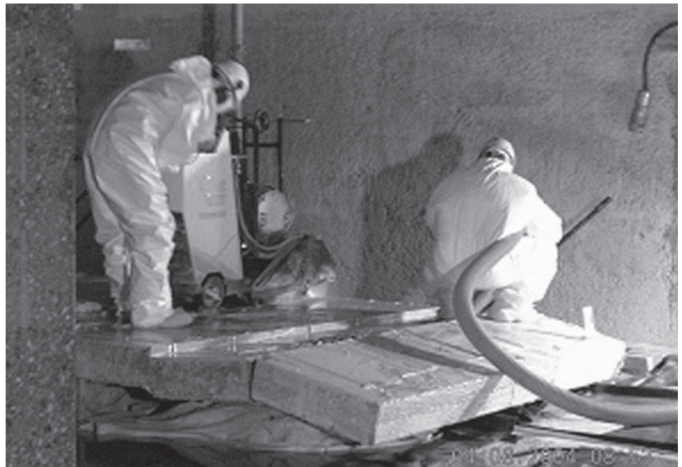
Figure 16: Workers Cut Contaminated Concrete from Building 771’s ‘Infinity Room’
