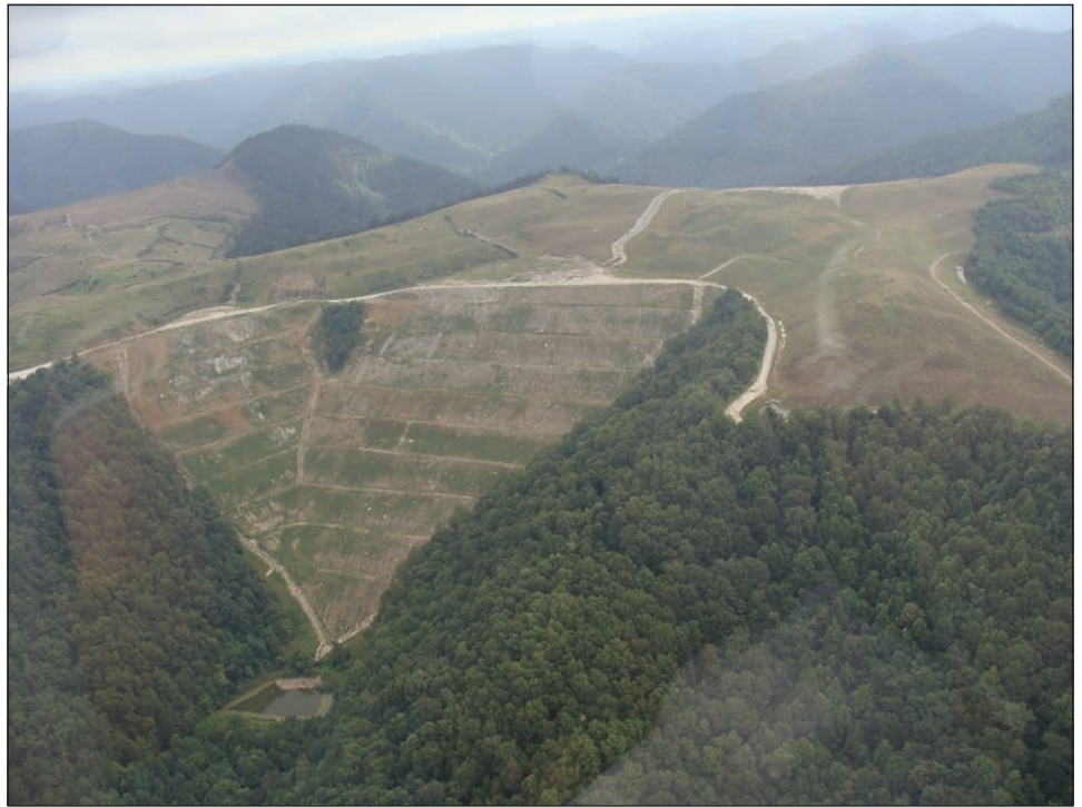
Figure 23: A Terraced Fill on a Reclaimed Site in West Virginia
