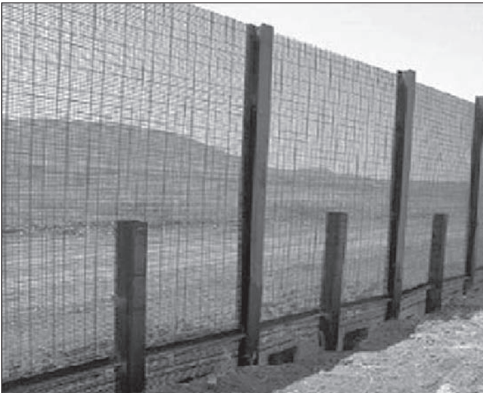
Post-and-rail fence with wire mesh
