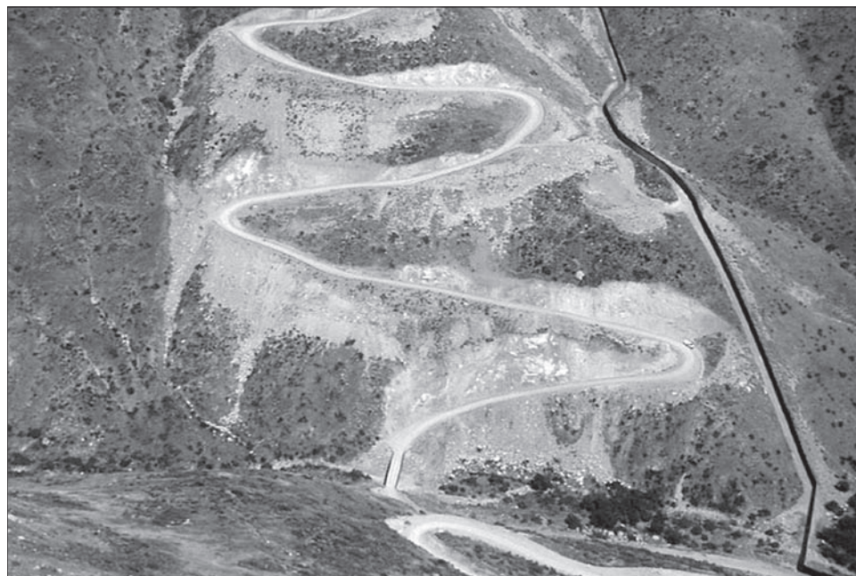
Figure 12: Fencing Project in Otay Mountain Wilderness Area, California, for Which DHS Is Providing Funding to Mitigate the Loss of Endangered Species Habitat
