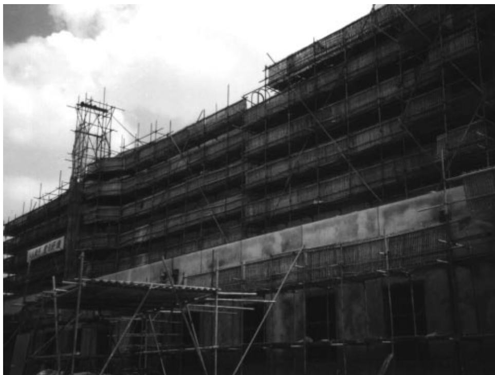
Figure 3: Machining Center Under Construction at the Shanghai Aviation Industrial Corporation
