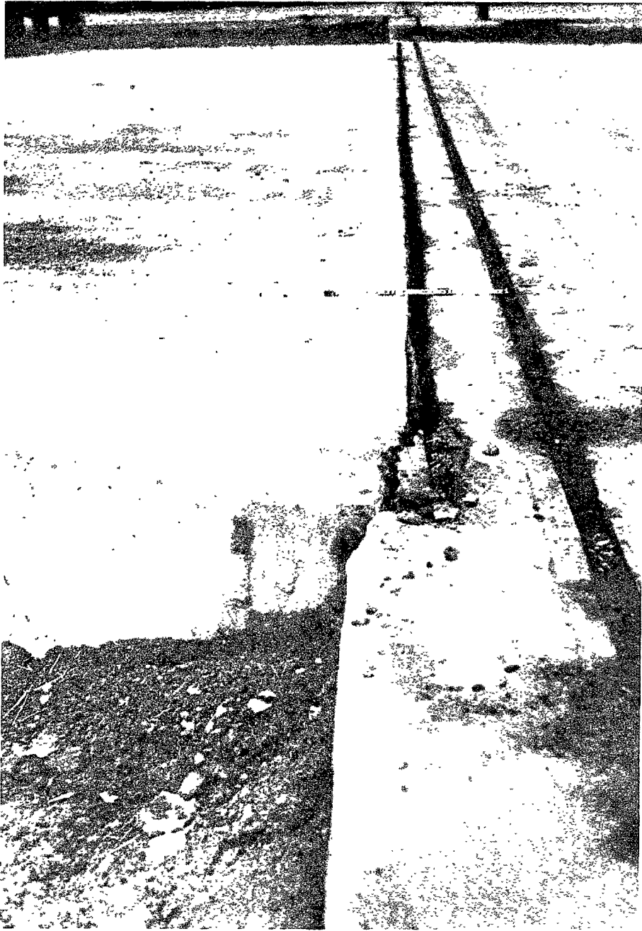
Photograph furnished by Ohio State Highway Department
