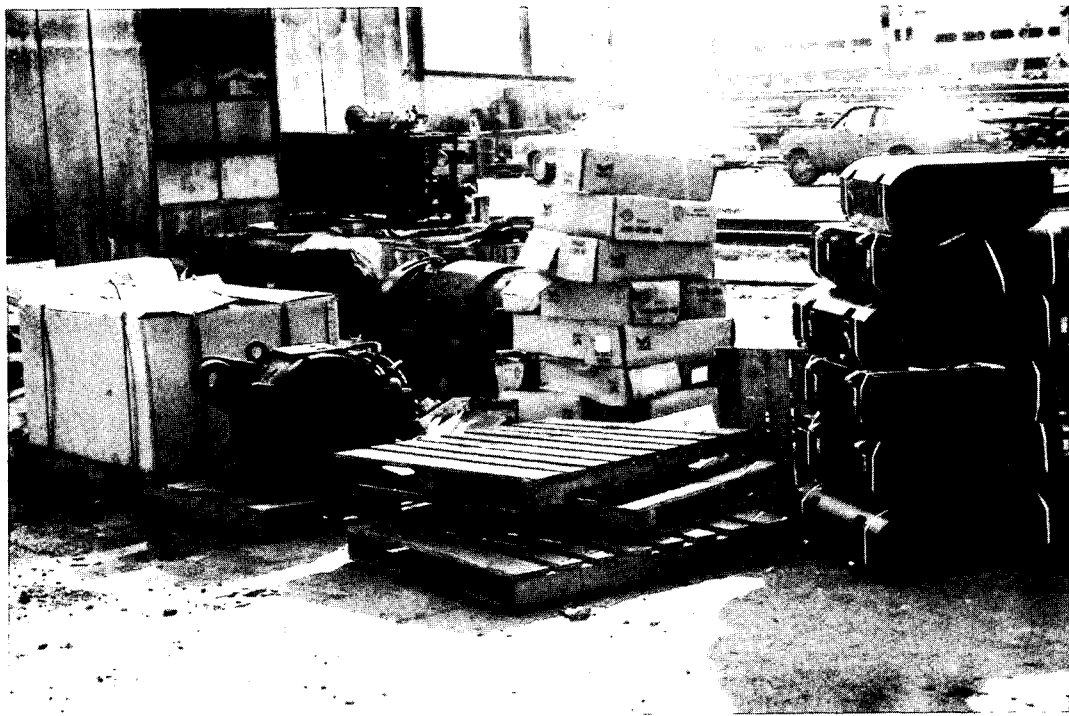
OUTSIDE STORAGE AT AMTRAK'S SUNNYSIDE, N.Y., MAINTENANCE FACILITY
