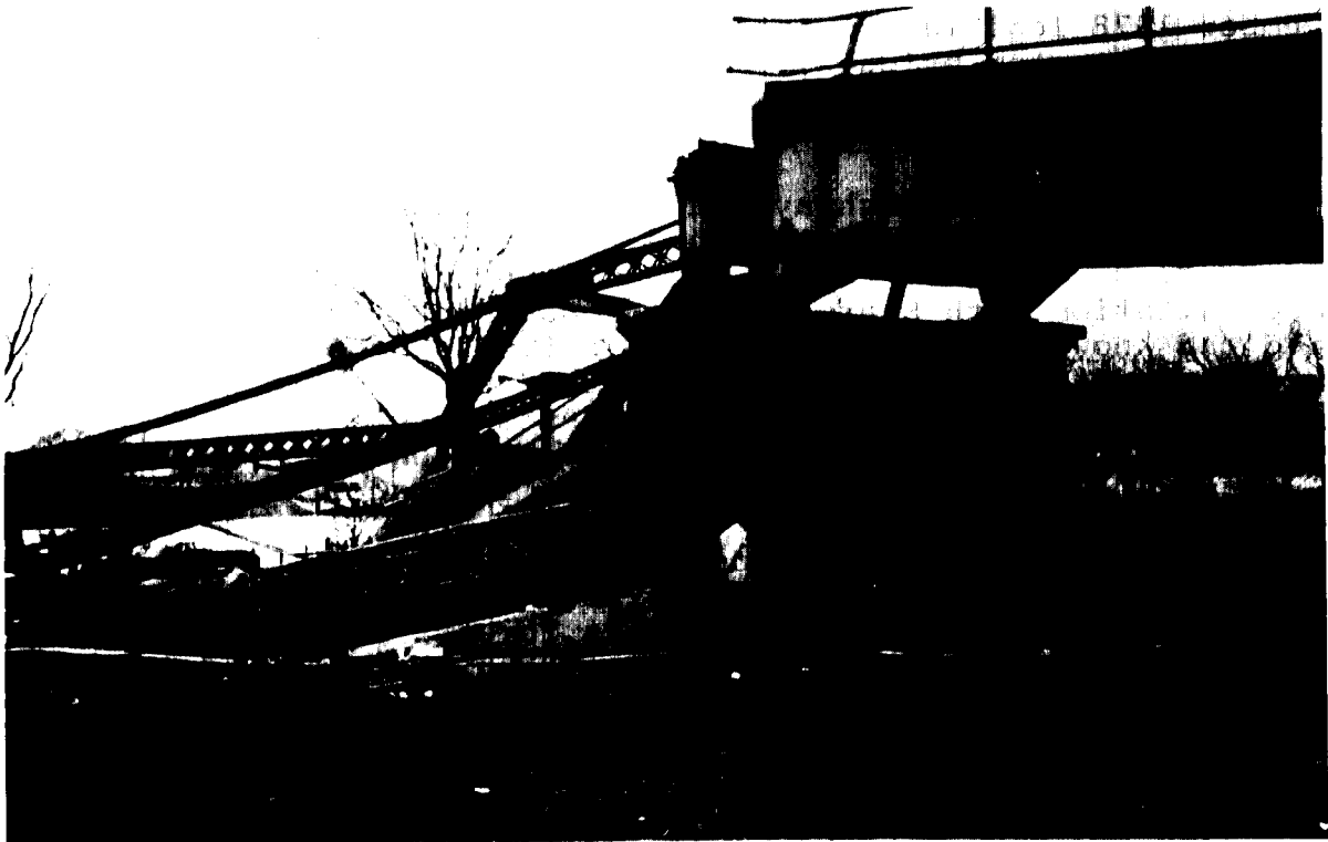
THE SILVER BRIDGE AFTER ITS COLLAPSE IN DECEMBER 1967. PHOTOGRAPHS COURTESY OF THE FEDERAL HIGHWAY ADMINISTRATION
