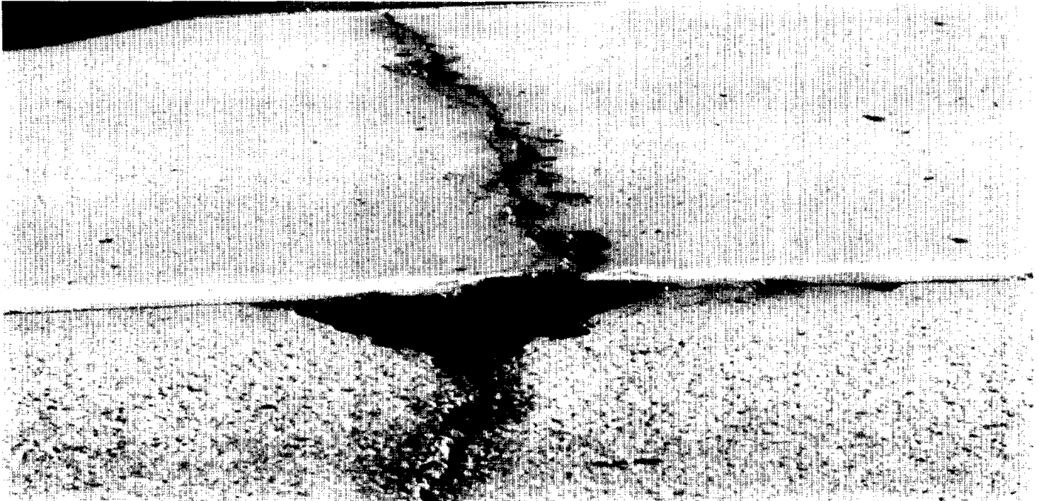
Figure 1.1: Distress Caused by Traffic
