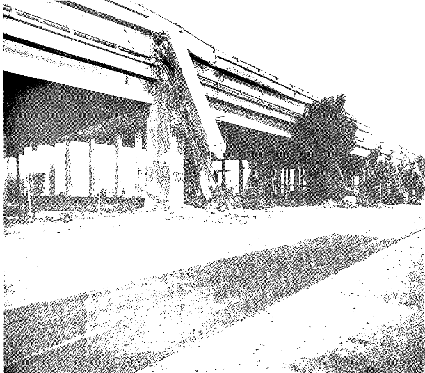
Figure I.4: Cypress Viaduct After October 17, 1989, Collapse
