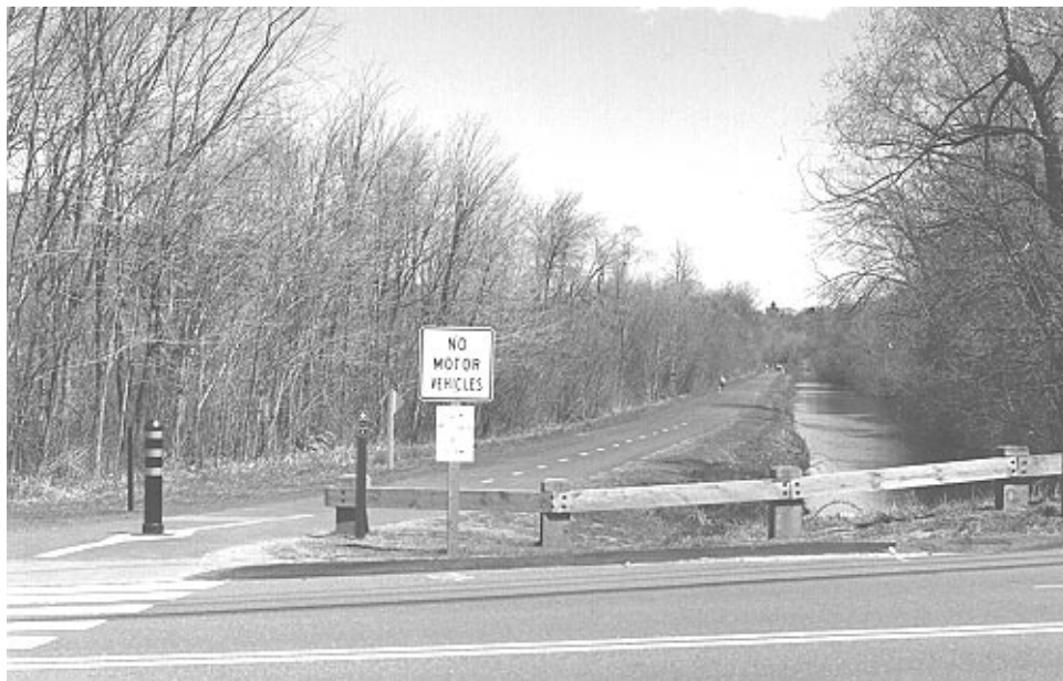
Figure VI.4: Site After the Railroad Right-Of-Way Was Converted to a Trail in Cheshire, Connecticut
