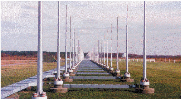
Relocatable Over-The-Horizon Radar (Receiver site antennas)
