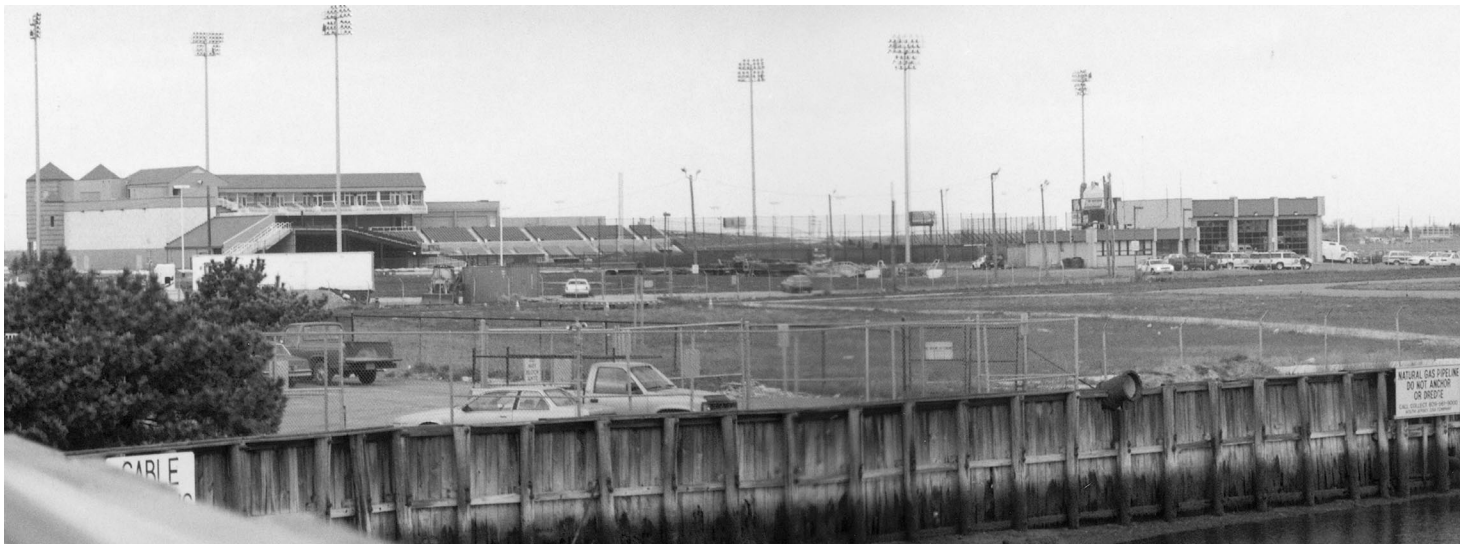
Minor league baseball stadium surrounded by floodlights. Atlantic City Police Department annex on the right behind the airport runway.
