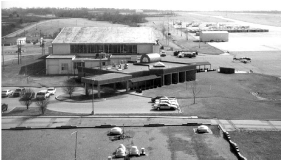
View of the terminal building (front) and aircraft hanger (back) and aircraft parking ramp.
