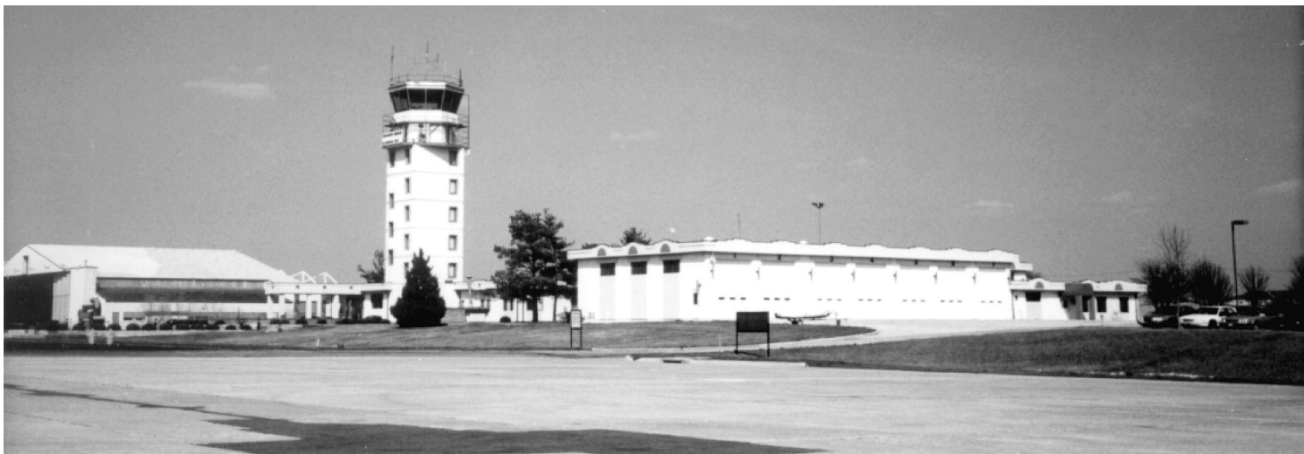
Air traffic control tower, parking area, and hangers.
