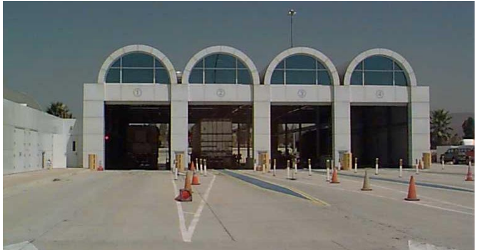
Figure 3: California State Truck Inspection Facility at Otay Mesa With Covered Inspection Bays
