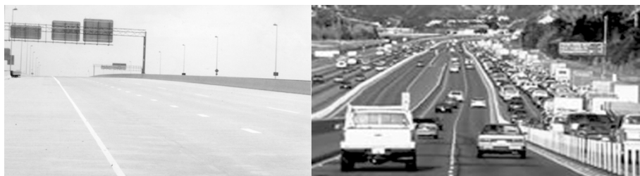
Sources: GAO (left); Orange County Transportation Authority (right).
