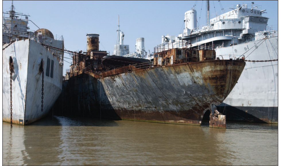
Figure 4: A High-Priority Ship Awaiting Disposal in the James River Fleet
