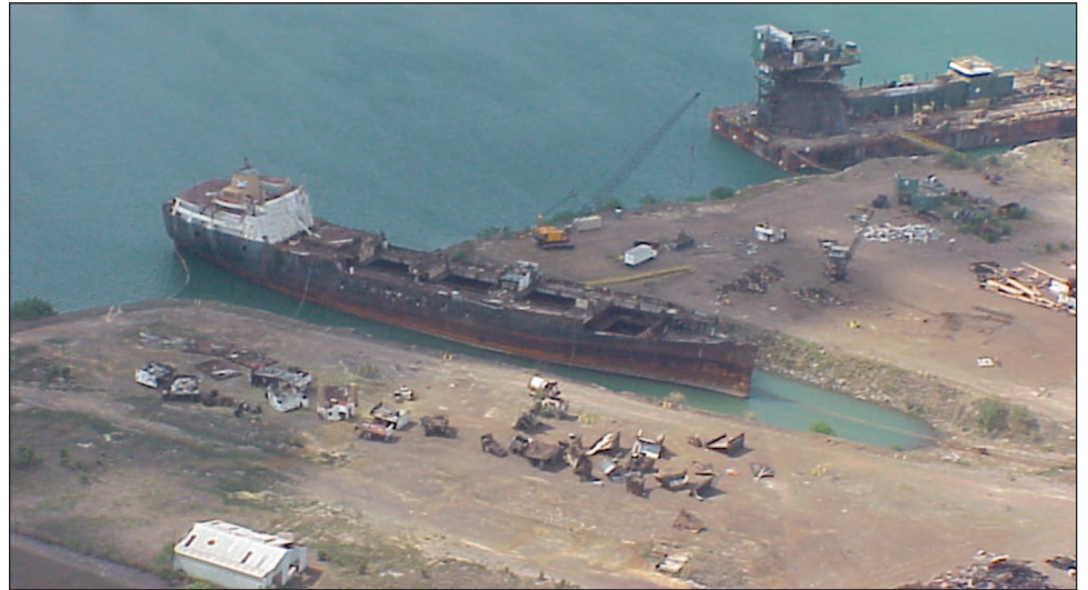
Figure 1: Ship during Early Stages of the Scrapping Process
