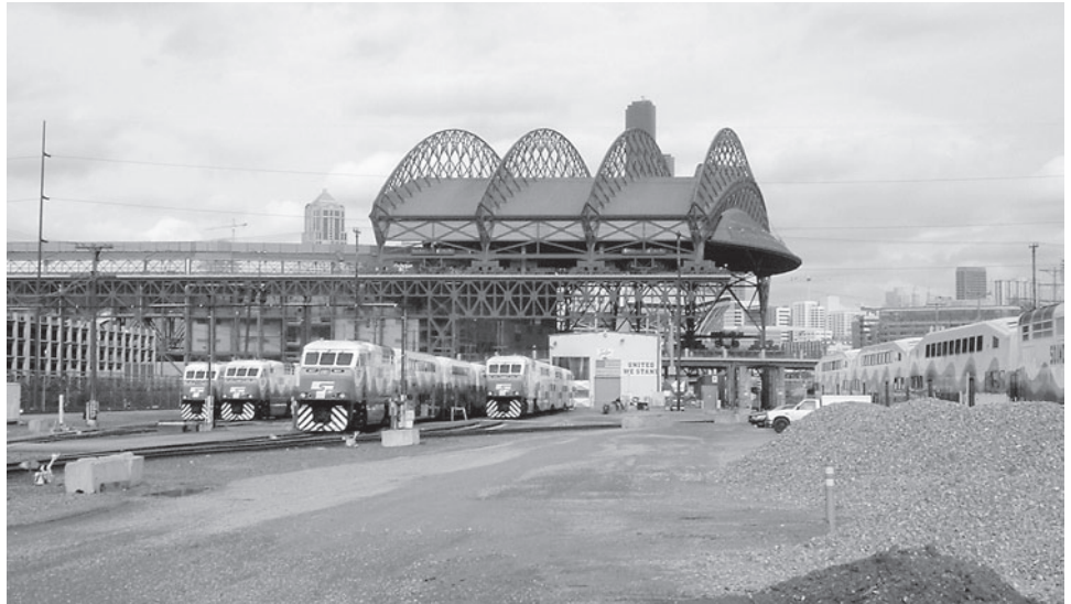
Figure 4: Sound Transit Trains in Amtrak's Holgate Yard, Seattle, WA
