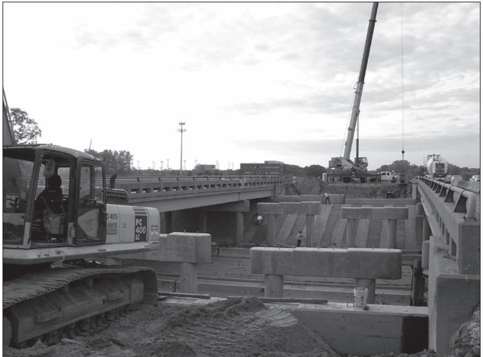
Figure 1: Recovery Act-Funded Pavement-Widening Project on M-59 near Detroit
