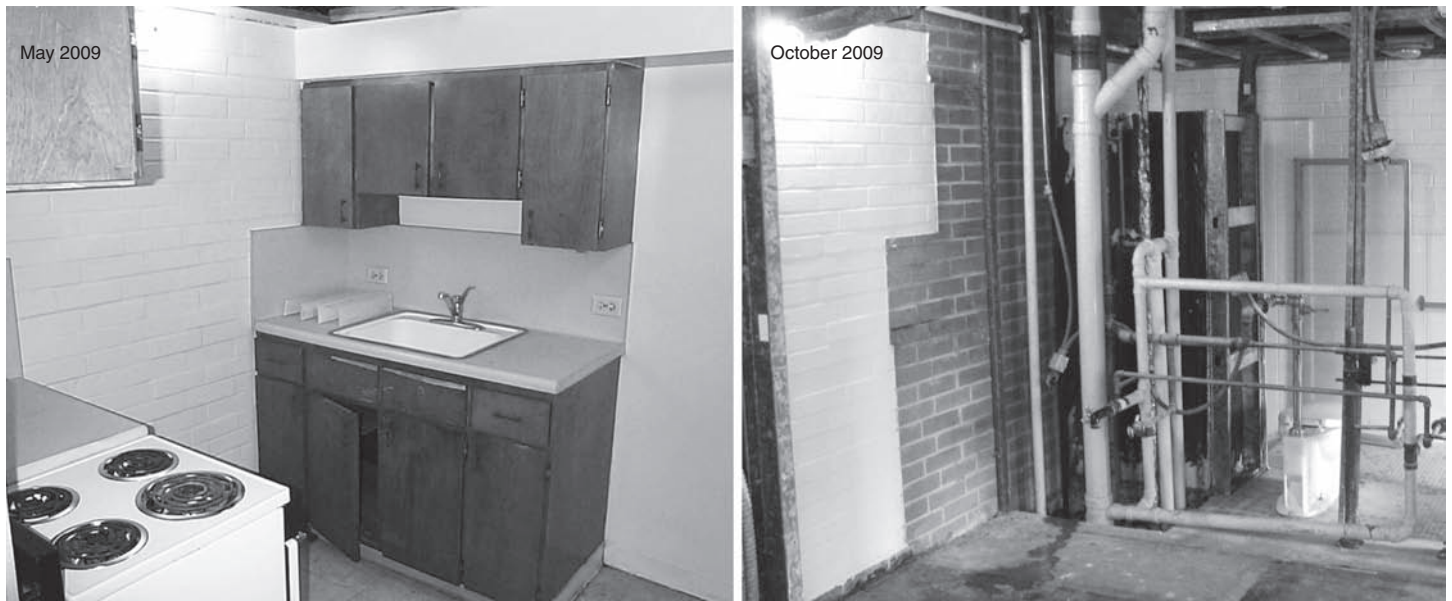
Figure 6: SAHA Unit Undergoing Asbestos Abatement
