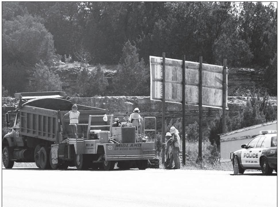
Figure 2: Resurfacing Work in Progress near Lago Vista, Texas
