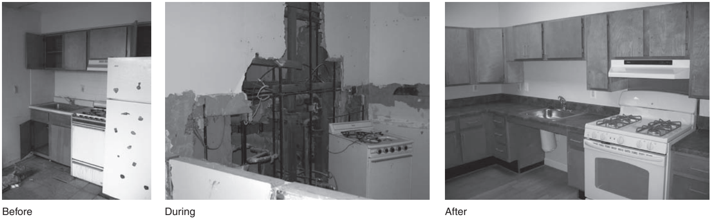
Figure 3: Kitchen Renovation at the Horizon House Public Housing Community
