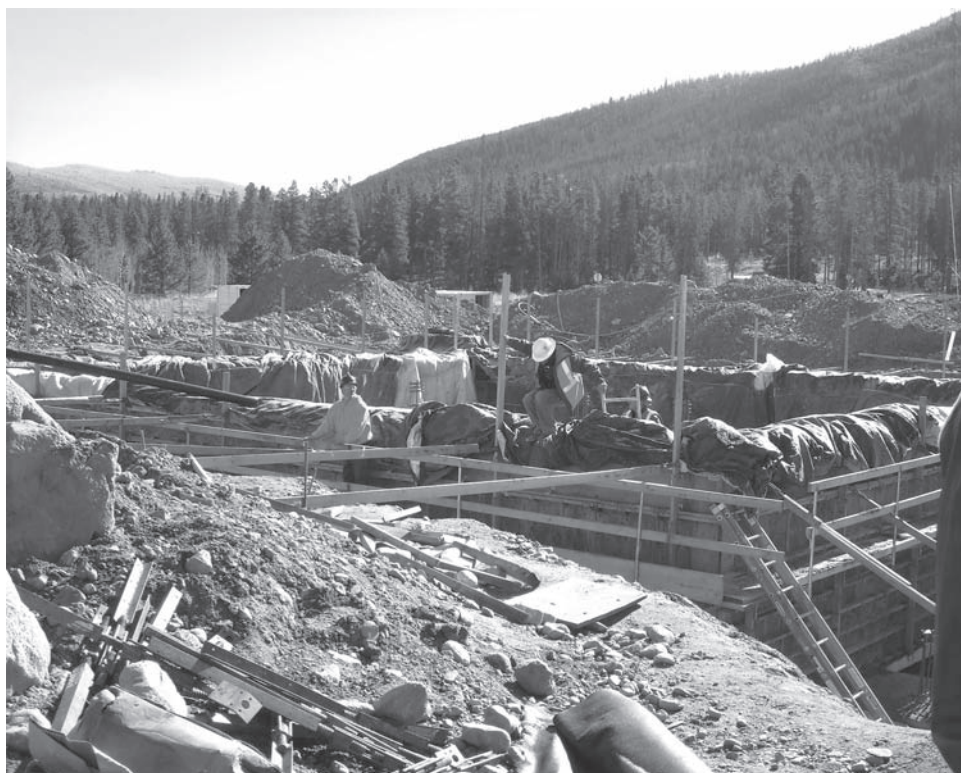
Figure 1: Summit County Bus Maintenance Facility under Construction
