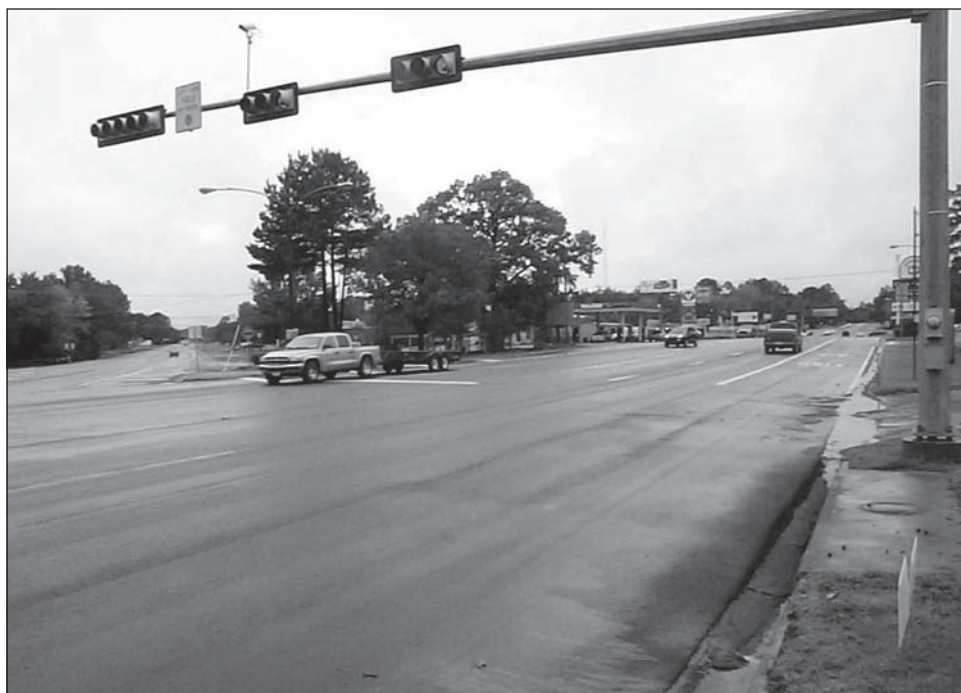
Figure 3: Completed Resurfacing Work in Mineola, Texas
