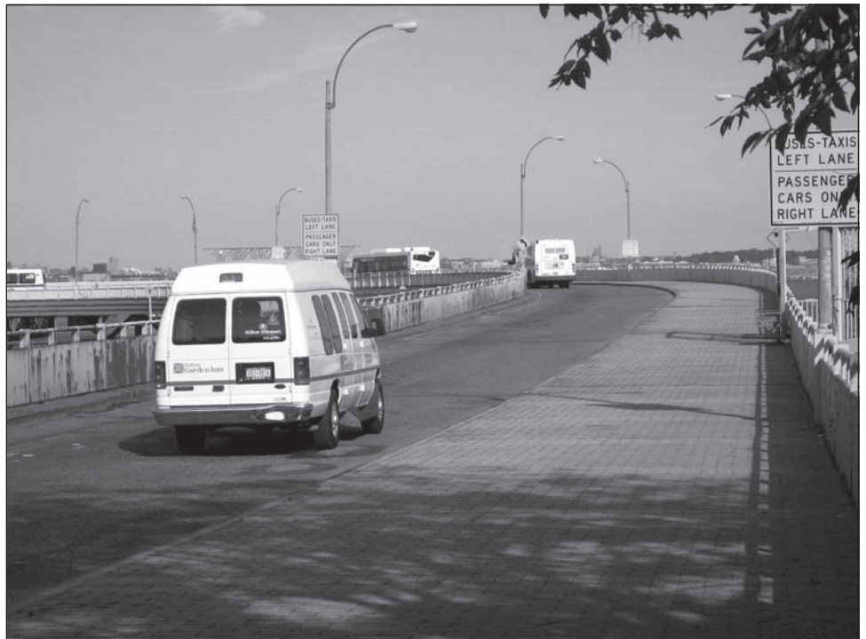
Figure 1: One of the Ramps That Will Be Rehabilitated at the St. George Ferry Terminal Using Recovery Act Funds
