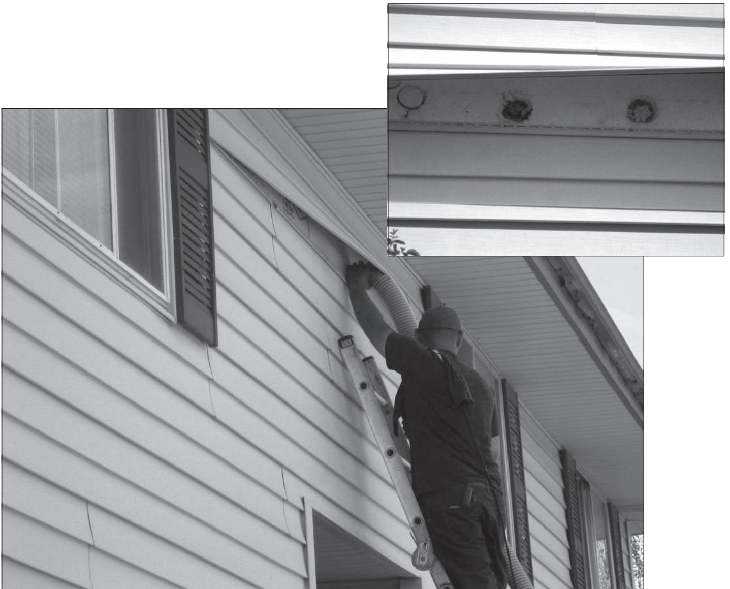
Figure 1: Arapahoe County Weatherization Worker Installing Insulation at a Home in Aurora, Colorado
