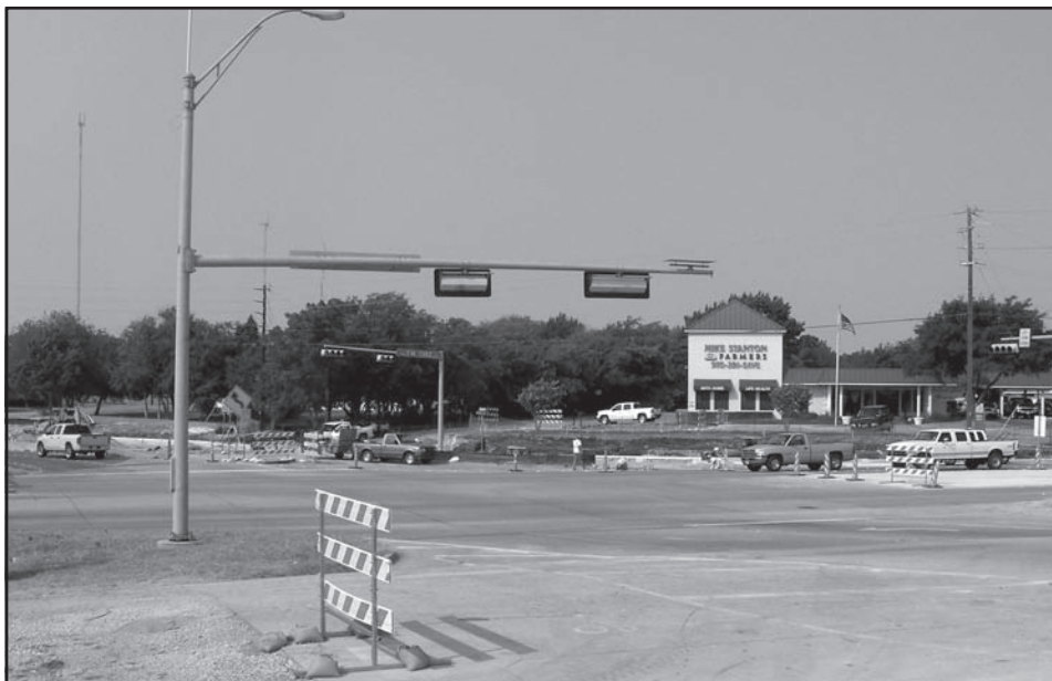
Figure 8: Cedar Hill, Texas, Intersection at Farm-to-Market Road 1382 and Straus Road, Temporary Turn Lane Constructed as Recovery Act–Funded Improvements Advance
