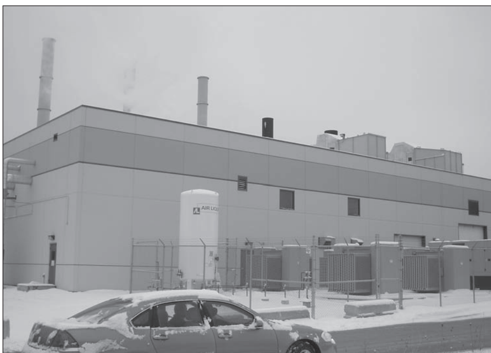
Figure 6: Energy Center Located at North Chicago Medical Center
