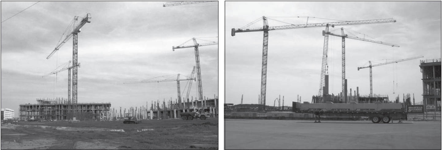
Figure 4: Ongoing construction of Orlando VA Medical Center, Florida
