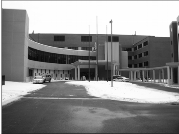
Exterior of the ambulatory care center at the Captain James A. Lovell Federal Health Care Center (FHCC)
