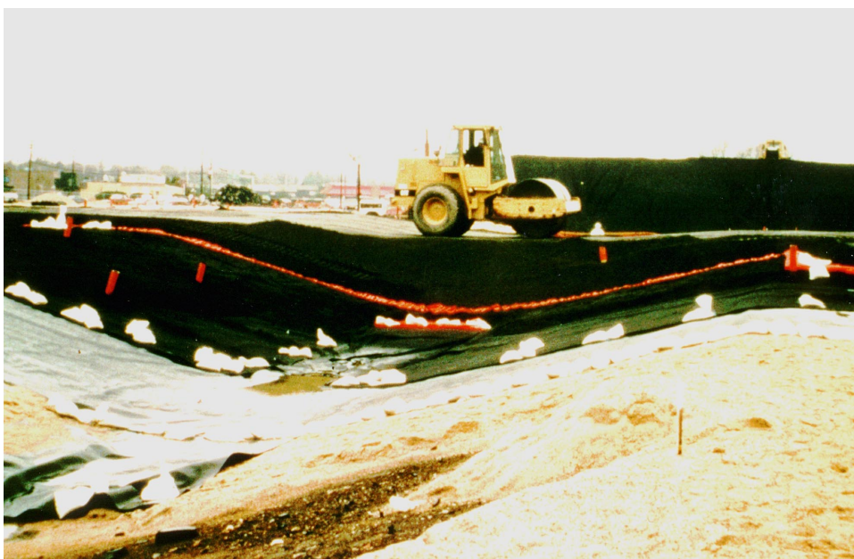
Figure 5: Construction of the Raymark Cap
