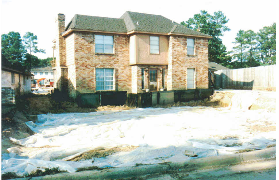
Residential Yard During Excavation
