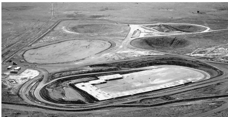
Figure 4: Disposal in Subsidence Craters at NTS and Mixed Waste Disposal Trench at Hanford
