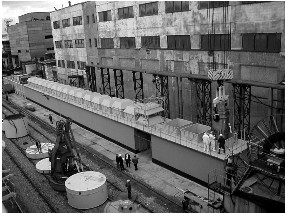
Figure 4: Interim Storage Pad
