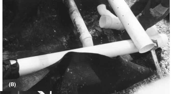
(B) Shows perforated 8-inch drainpipes (PVC schedule 40) used for the drainage system being installed under the concrete mud mat. The drainpipe is wrapped with a permeable filter fabric and buried in gravel, and an impervious filter fabric is then laid on top to keep out silt and dust. The mud mat is poured on top of the gravel base.
