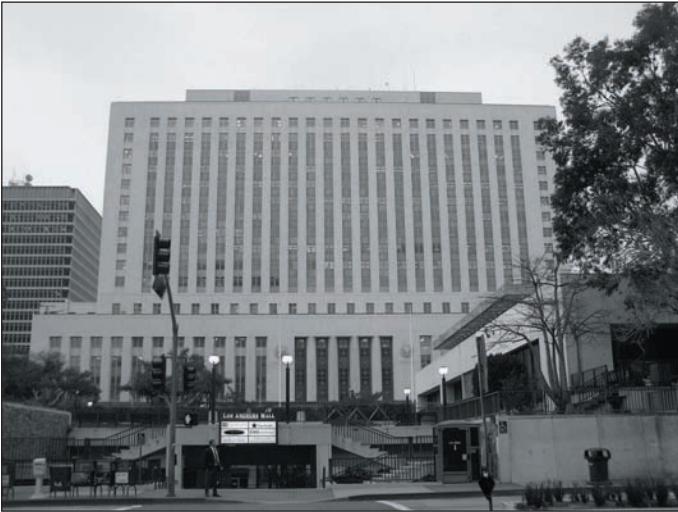
Figure 1: U.S. District Courthouses in Los Angeles
