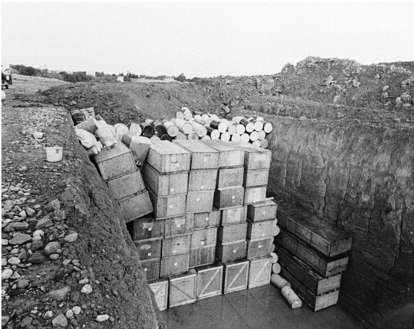
Figure 2: A Trench in the State-Licensed Disposal Area During Past Operations
