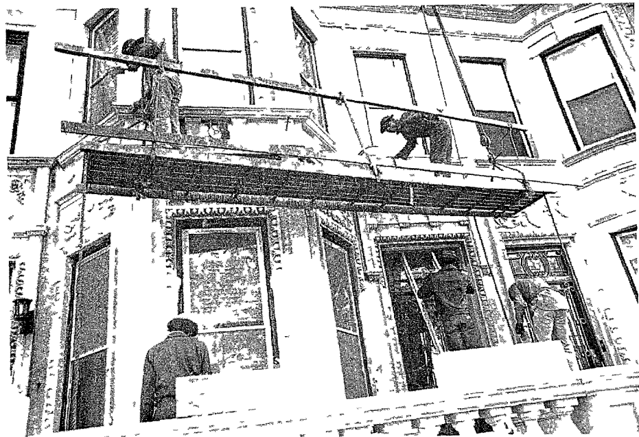
EXTERIOR RENOVATION WORK
