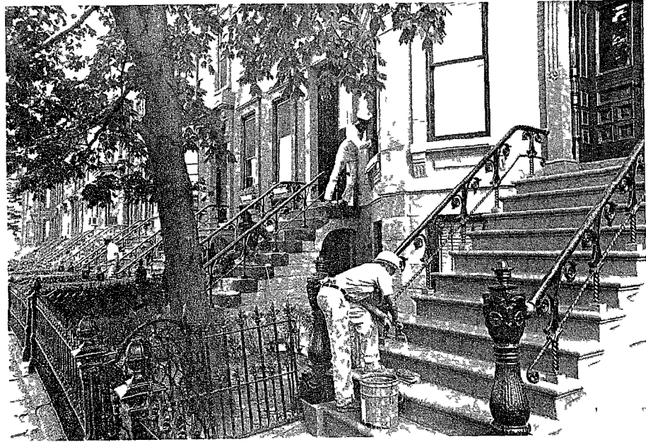
EXTERIOR RENOVATION WORK
