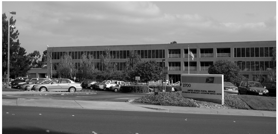
Figure 1: The San Mateo IT Center
