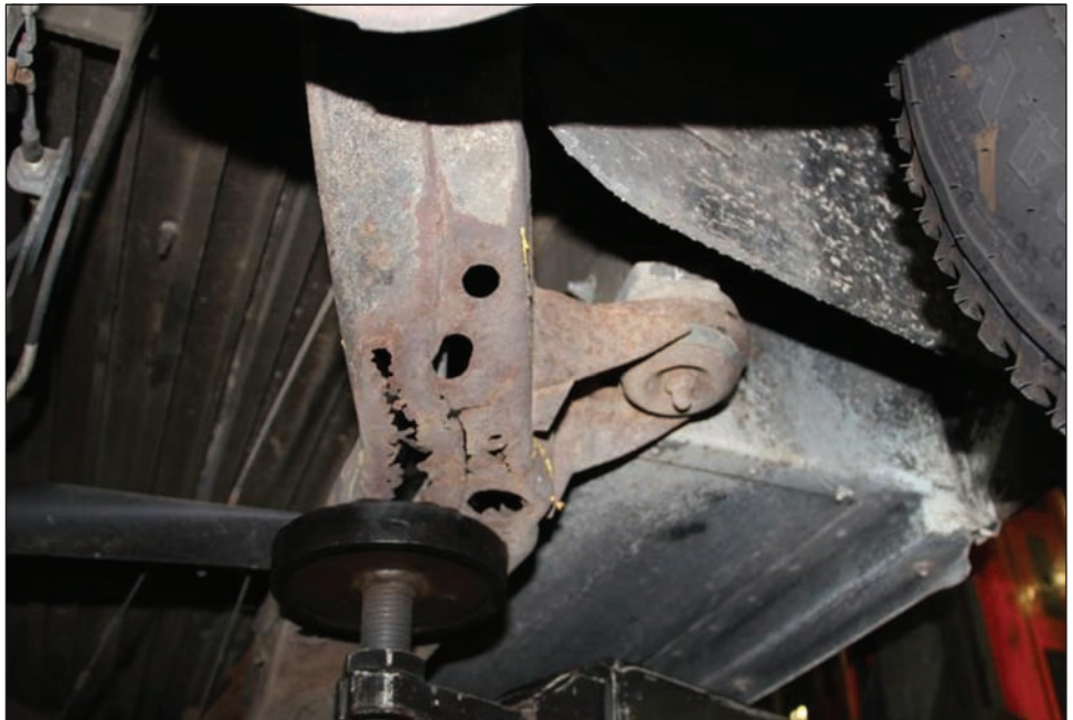
Figure 11: Rusted Frame with Holes Being Replaced in a USPS Vehicle Maintenance Facility in New York State, 2010
